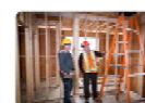
Construction Reduction of falls from heights — with a particular emphasis on falls from ladders.
